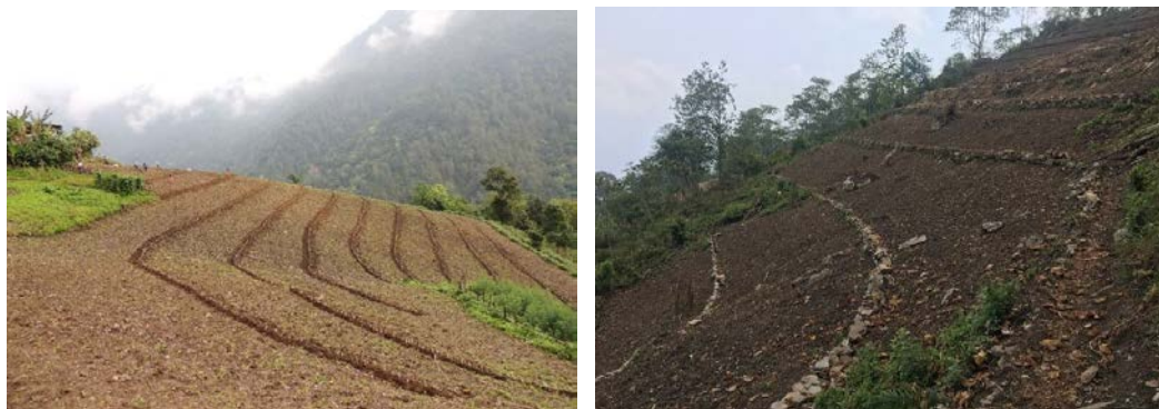
Figure 10. Land Terracing (L) and Stone Bunding (R)
