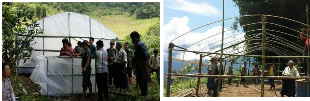
Figure 16. Low-cost poly-house using bamboo frames
