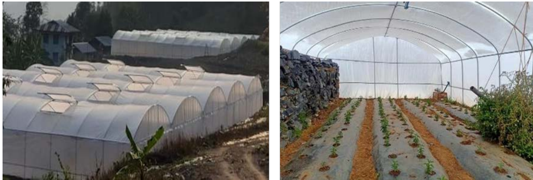
Figure 8. Mega Greenhouse Structure
