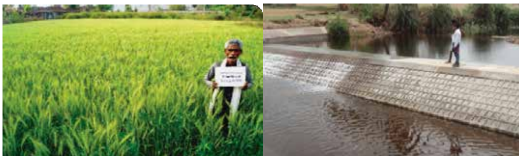
Fig. 1 Construction of check dam in Chitrakoot district of Bundelkhand region
