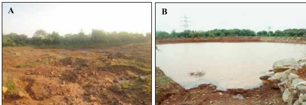
Fig. 3 Community Pond before desilting (A), and after desilting (B)
