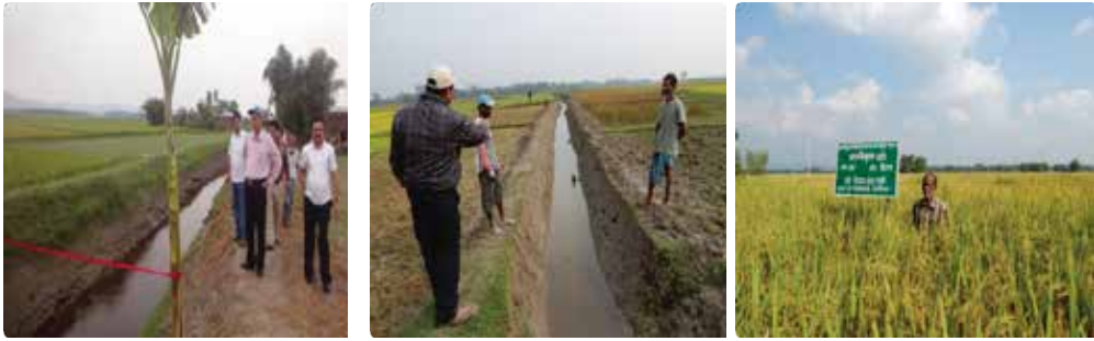
Fig. 21 Desilting of drainage channel in Dhubri district of Assam
