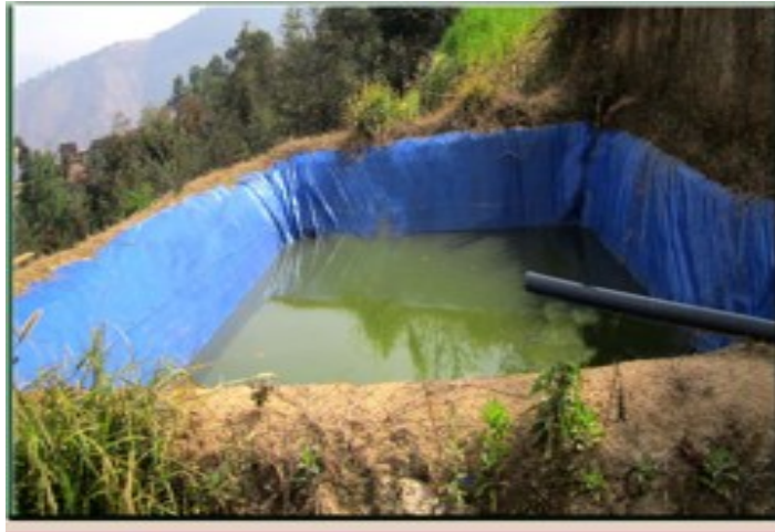
Fig. 17. Rainwater harvesting plastic pond
