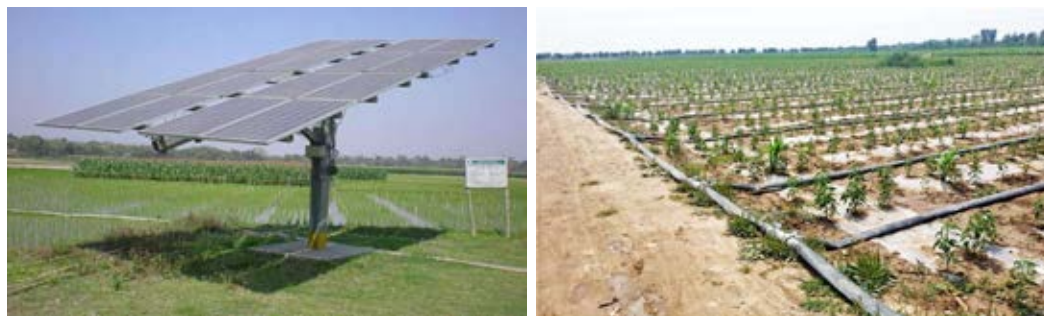
Fig. 5. Field irrigation by using the solar water pumping system
