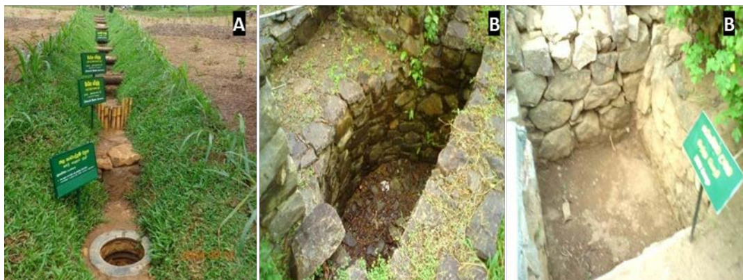
Fig. 31 Percolation pits (A) and Silt trap (B)
